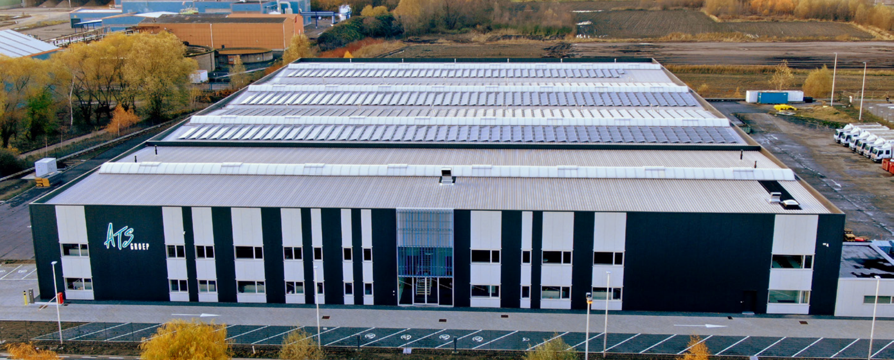
Demosite 'Smart Buildings' ATS Langerbruggekaai Gent.
